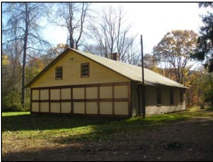
Civilian Conservation Corps structure in Croyland
