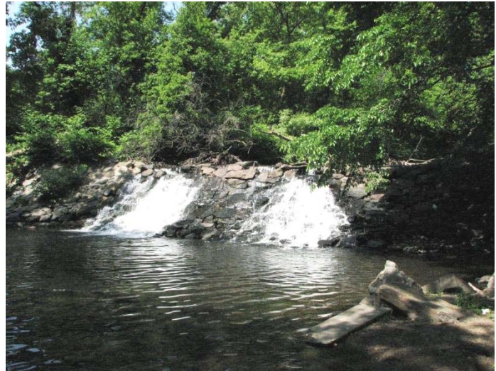
Millbourne Dam, a run-of-the-river dam, across Cobbs Creek between Philadelphia and Delaware County.
