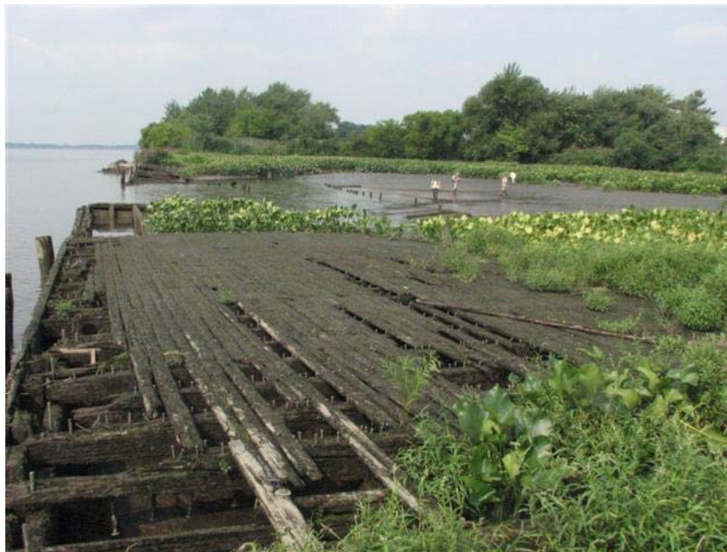
The abandoned wooden pilings, piers and ramps within the river help to diminish the impact of wave action from passing ships on the river shoreline and may help to encourage the formation of tidal mudflats along this portion of the river.
