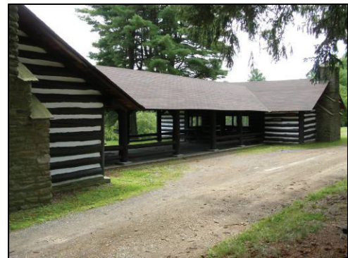
Cherry Springs State Park Picnic Pavilion built by the Civilian Conservation Corps
